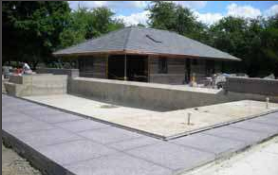
Granite pavers installed on a pedestal system allow water to flow through the open joints and into a hidden channel drain in the pool deck.
